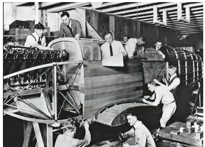
Douglas Cloudster under construction
